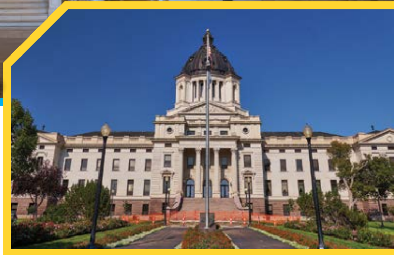
South Dakota State Capitol Building in Pierre
